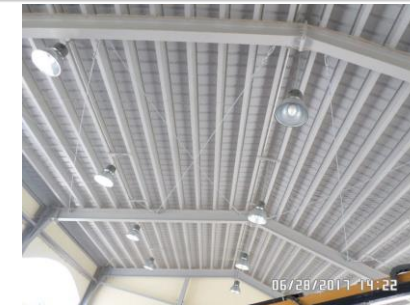
Figura 3 – Vista interior do teto. Figure 3 – Interior view of the roof.
