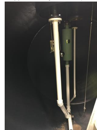
Figura 5 – Interior do tanque Figure 5 – Tank interior.
