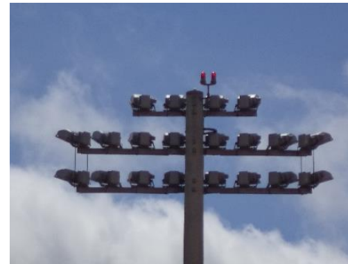
Figura 1 – Instalação de novos holofotes. Figure 1 – Installation of new floodlights.
